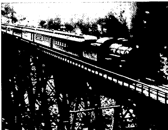
Utah's railroad construction included trestles, tunnels, bridges, grading and track-laying.
