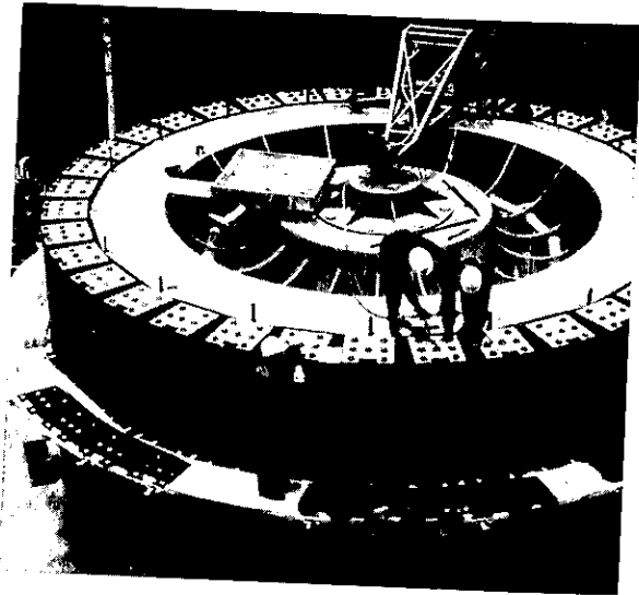
Canadian GE generator being installed at Labrador's Churchill Falls.
