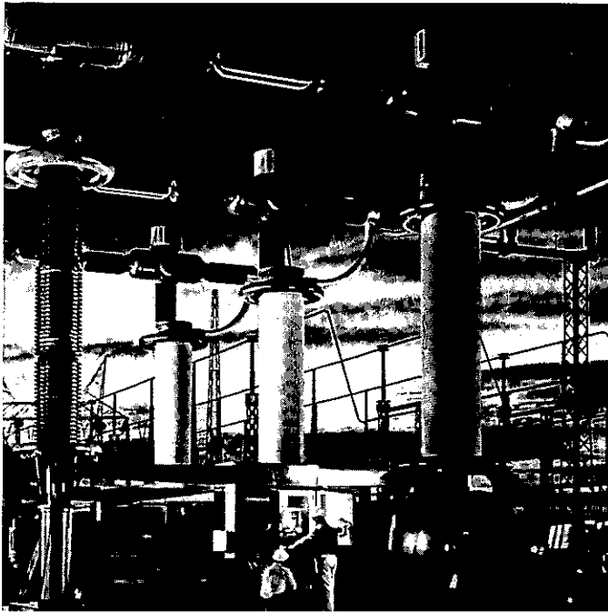
New 500-kv air blast circuit breakers protect Arkansas Power and Light EHV line.
