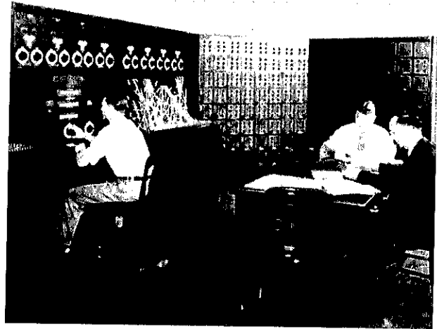
The ac network analyzer being used to solve a power company operating problem (1938).
