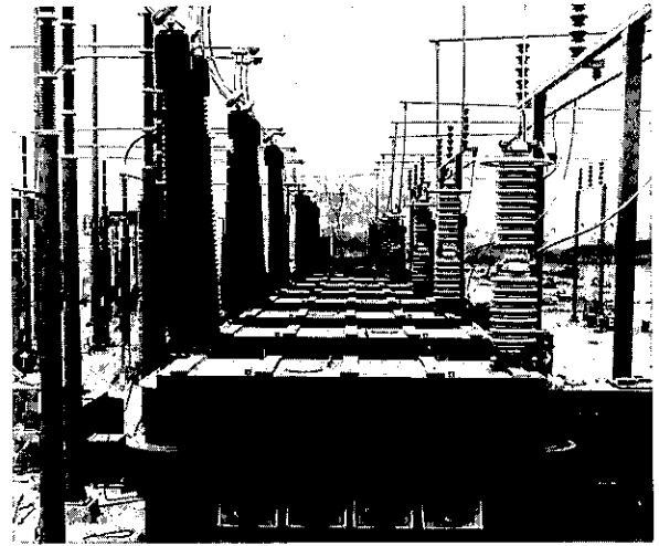
Transformers and power bushings for the Pacific HVDC Project on the Columbia River in Oregon.
