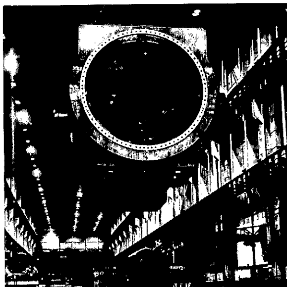
Portion of 260,000-kva generator with liquid-cooled stator.
