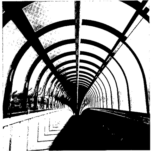
Lexan high impact resistance sheet used at rebuilt Yankee Stadium in New York City.
