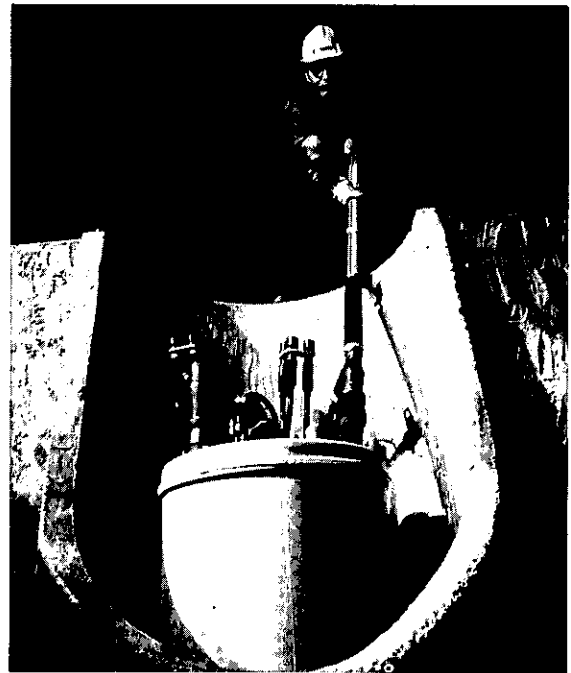
Underground distribution of power is more feasible with the development of new transformers.
